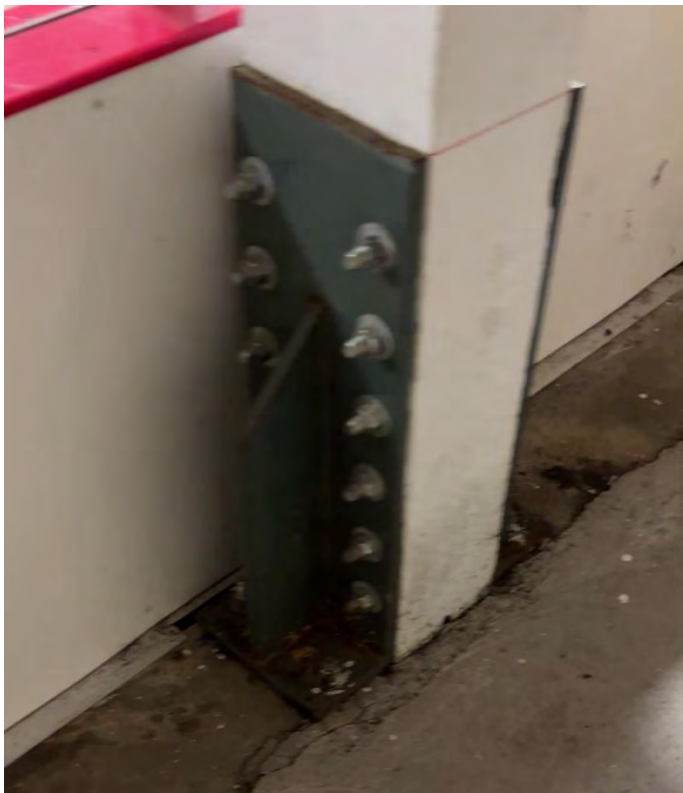
Photo: Steel Bracket Reinforcing
